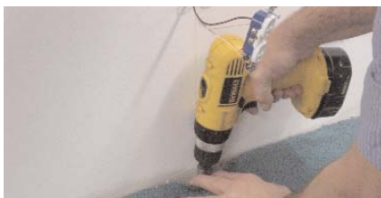
DRILL 1/2" HOLE PARALLEL TO WALL THROUGH FLOOR WHERE VERTICAL LINE FROM OUTLET MEETS FLOOR.
