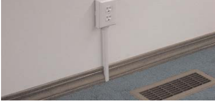
FINAL SURFACE WIRING INSTALLATION WITH ASLL.
